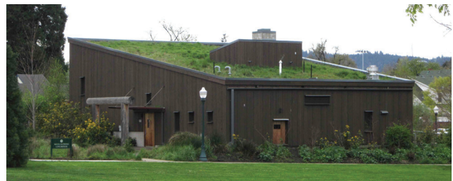
Many Nations Longhouse bioswale and green roof
